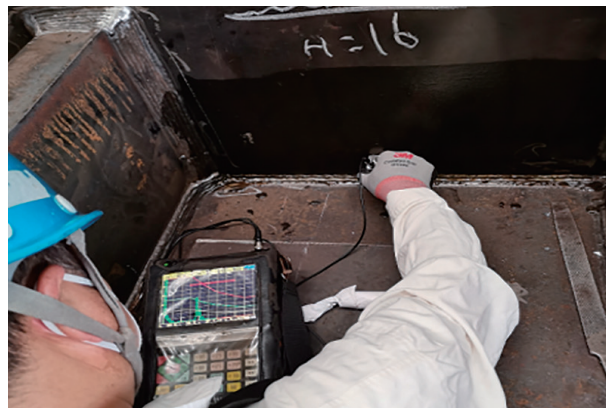
焊缝检测 / Weld Line Inspection
